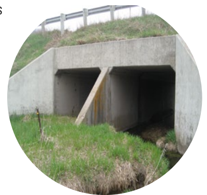
Culverts divert water along, under, and away from roadways to prevent flooding and make for safer travel..
